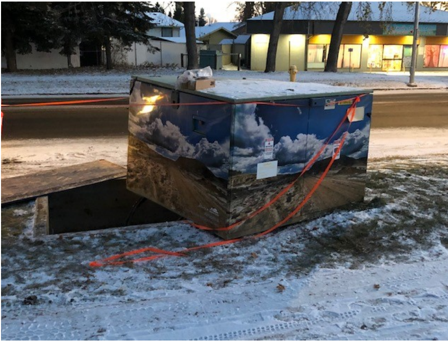
Top Left: The transformer box off of its mount on Oct. 20th
